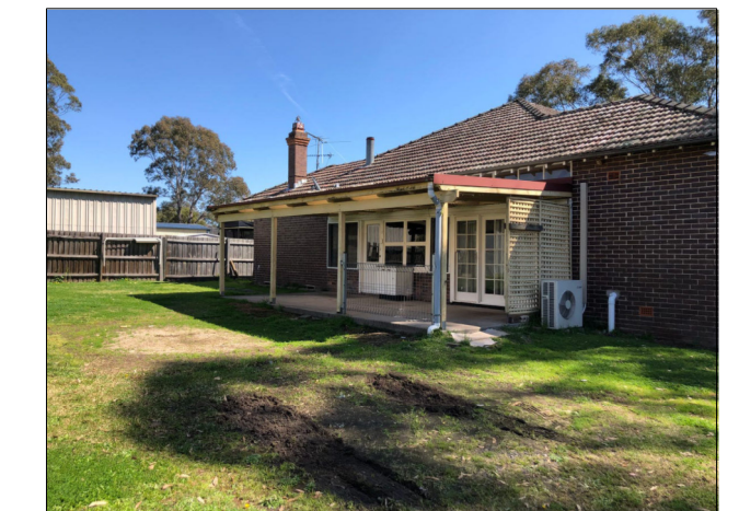
IMAGE 3 - External view of existing rear verandah
