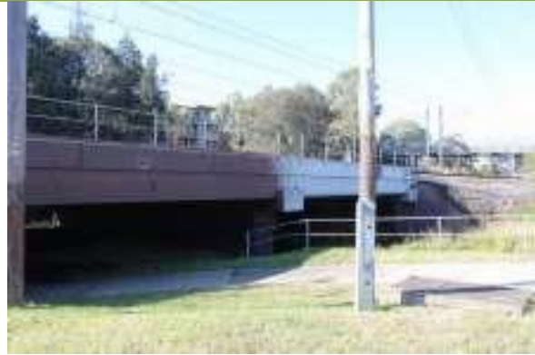
View east to Underbridge from Portico Parade
