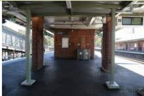
View north to Station Building on Platform 3/4.
