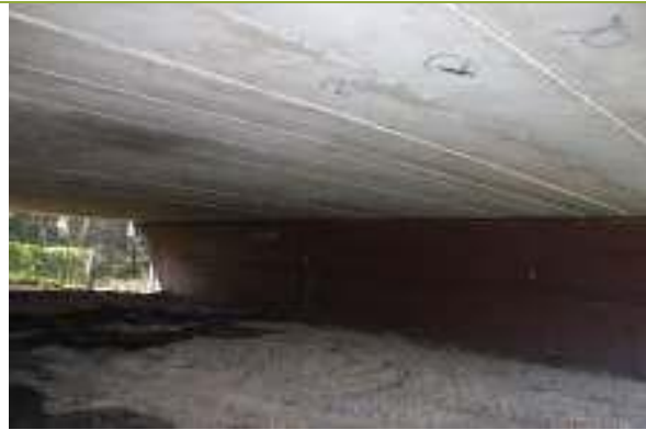
View south under contemporary underbridge, to location of archaeological remains
