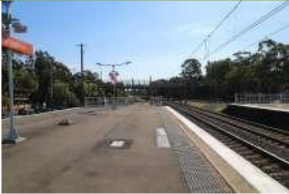
View north towards underbridge.
