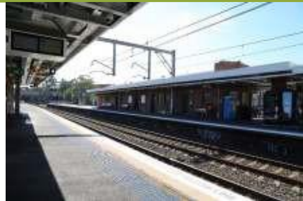
View from platform 3 to platform 2.
