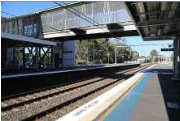
View southeast to Platform 2.
