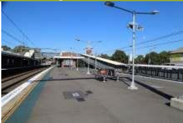
View south from platform towards concourse.
