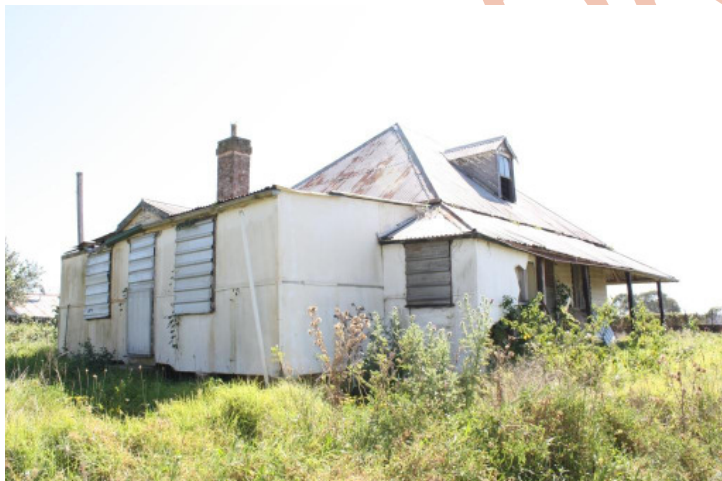
Figure 3: South eastern corner.
