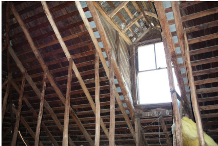
Figure 15: View of the uncut timber framing forming up the dormer roof.
