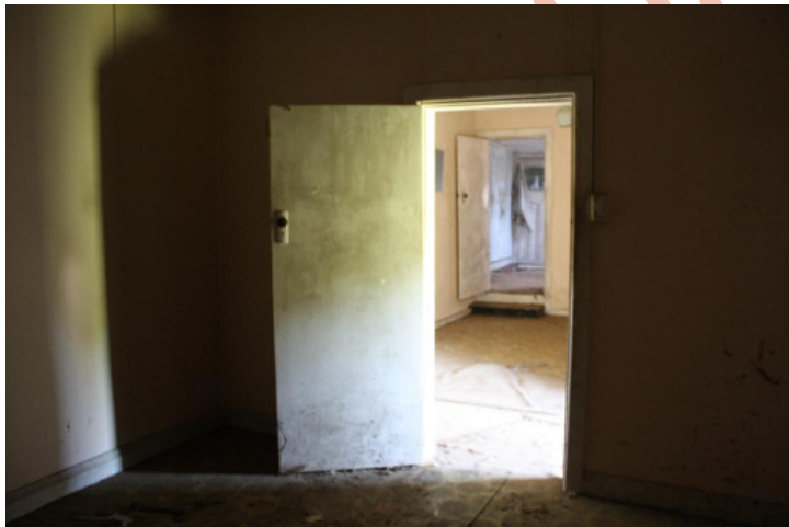
Figure 11: View through doorway of Space 6 across Space 5.
