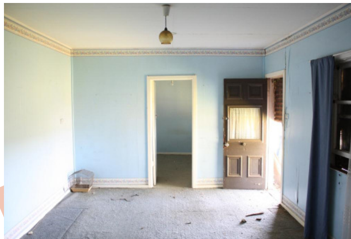
Figure 6: View across Space 1 towards Space 2.
