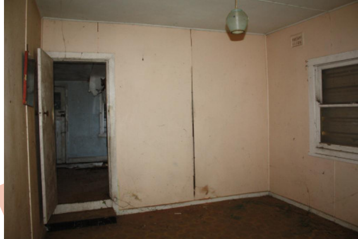
Figure 10: Space 5 - Fibre cement sheeting cladding the walls of Space 5.
