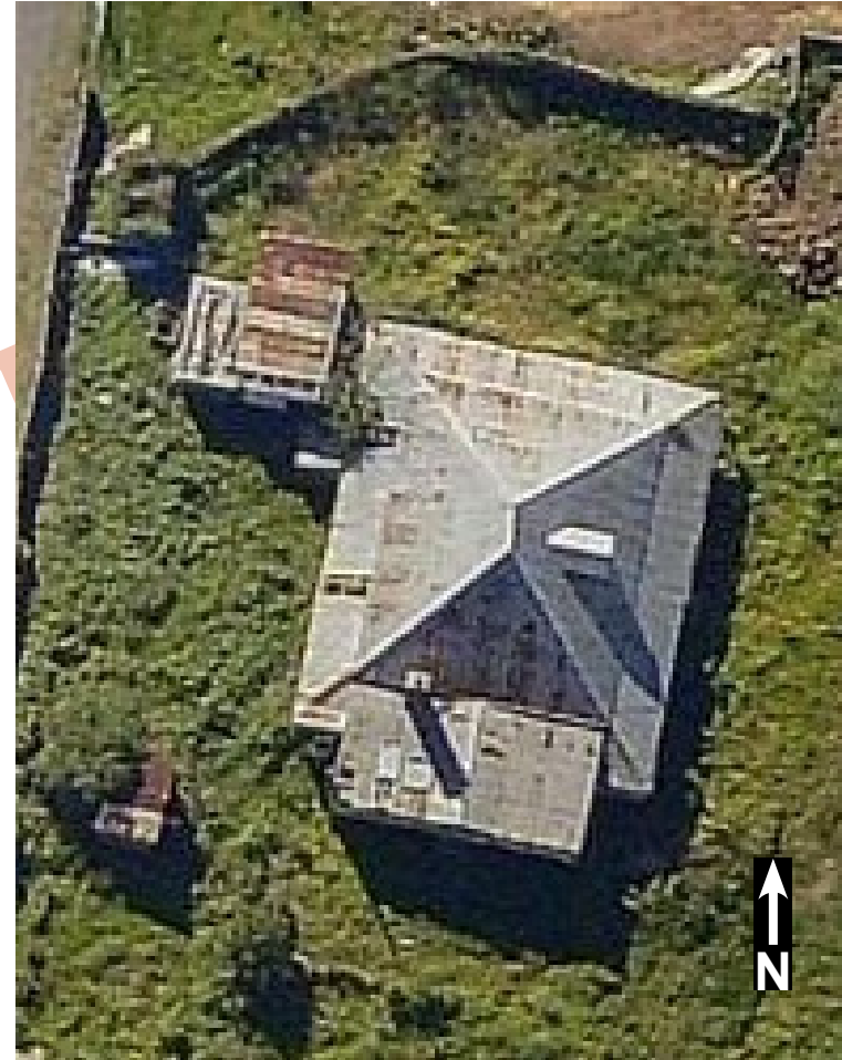
Aerial view of the Policeman's Cottage.
