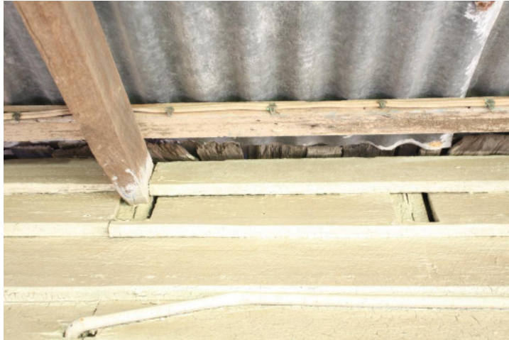
Figure 13: Detail showing exposed edge of earlier timber shingle roof.
