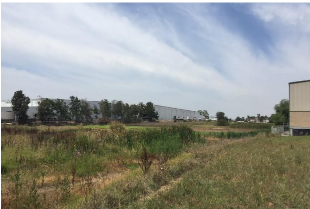
Figure 5 Adjacent Industrial Buildings (east)
